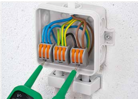
Testing the wired connectors
