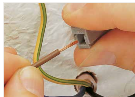
To remove: Press button and withdraw conductor.
