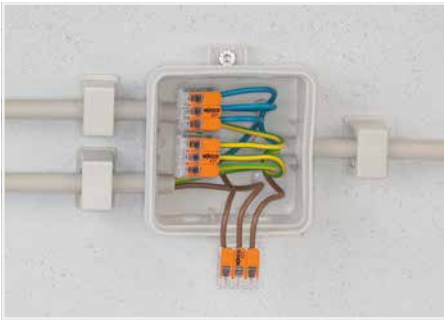
Wiring fine-stranded conductors in a junction box
