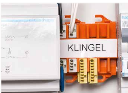
DIN-35 rail-mount application (residential door bell)
