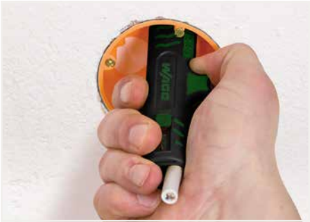
Stripping a cable sheath.
